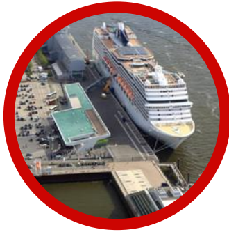
Onshore power supply facility in the Hamburg Cruise Center Altona
